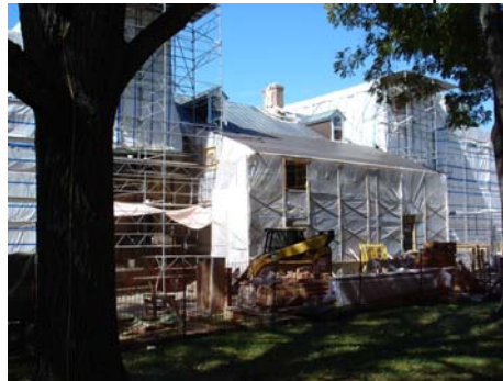
Montpelier under renovation
